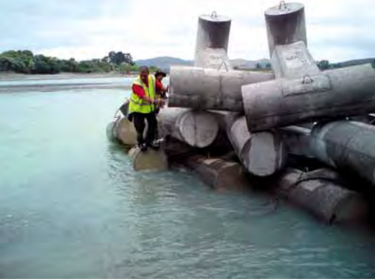
Above: Installation of dolosse.
