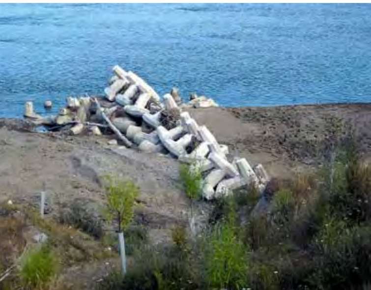
Above: Addition dolosse placed onto the groyne. The poles planted can be seen in the foreground.
