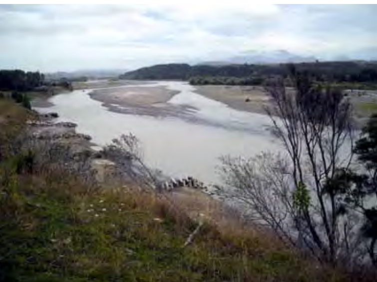
Above: Islands are forming behind groyne.
