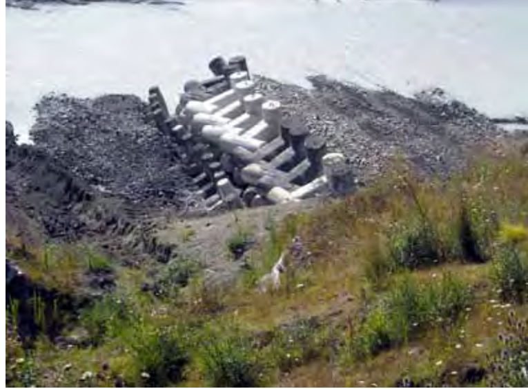
Above: Groyne being created on the Waiapu River.
