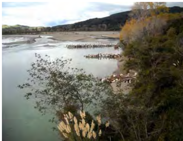
Above: Third groyne installed earlier this year.
